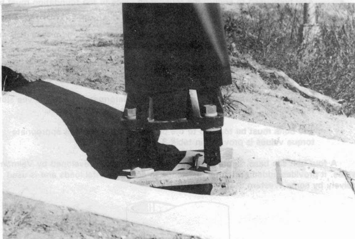
Figure 3.10.10 - Frangible coupling luminaire support
