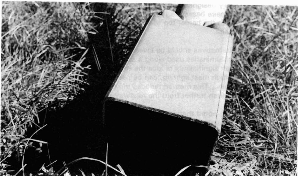
Figure 3.10.17 - Separation of bottom flange from T-base
