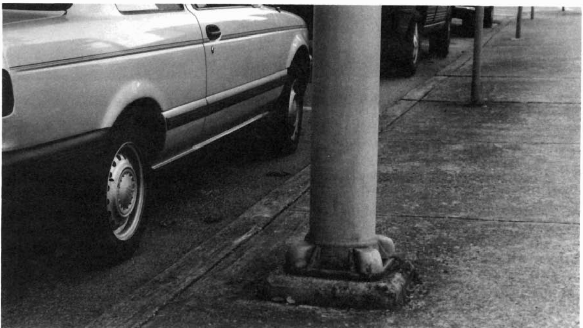
Figure 3.10.8 - Flange steel base
