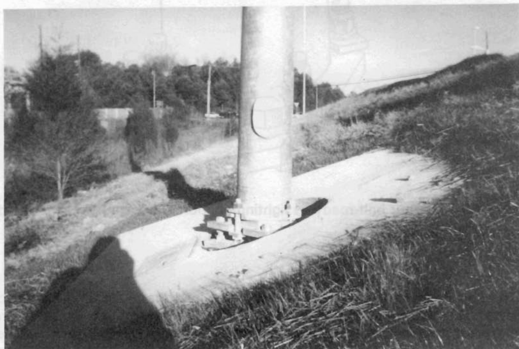
Figure 3.10.11 - Roadway lighting support slip base
